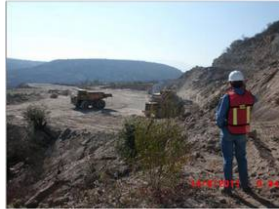
UNUSED MATERIAL LOAD AND HAULING
