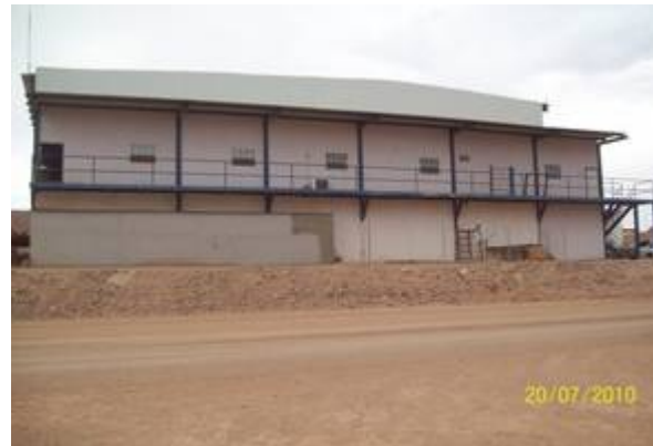
OFFICES BUILDING INSIDE THE MINE.
