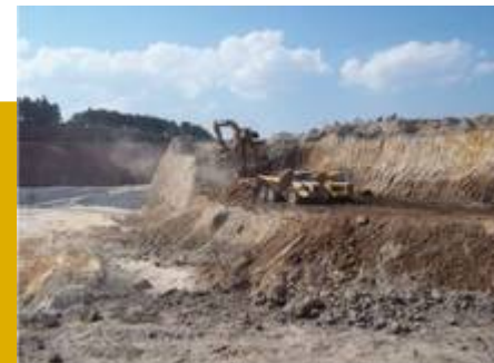
LOAD AND HAULING IN AHUAZOTEPEC
